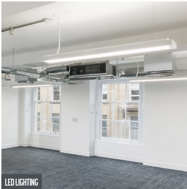
EXPOSED VRF AIR CONDITIONING
